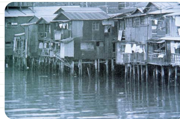
▲ Illegally constructed structures crowded the shores of the Murasakigawa River. Filthy water drained into the river.
